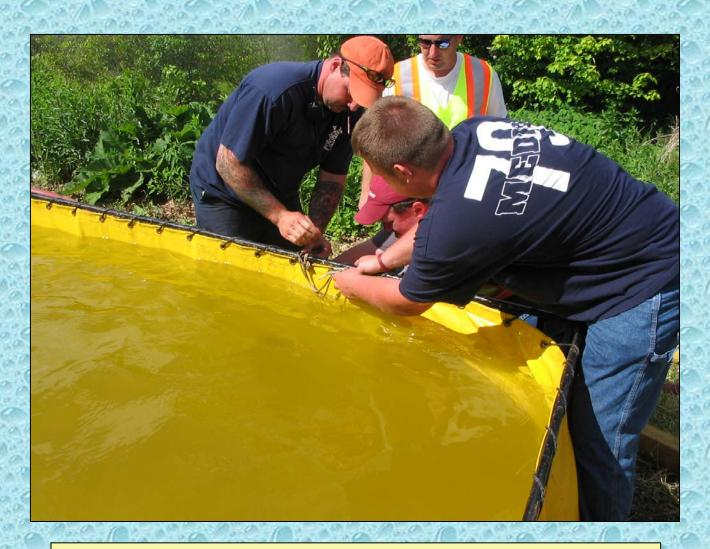
The position of dump tank drains when packing up after a call is really not important...until of course, the next call when the tank is filled with water.
