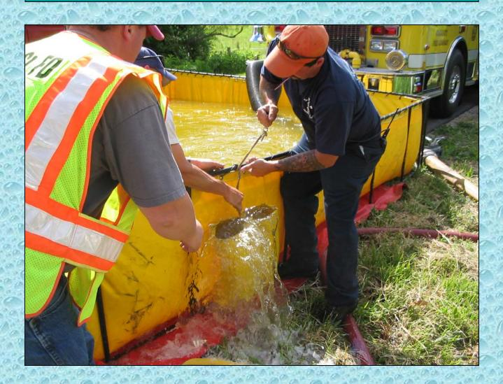
This drain was tied up on the outside of the tank when it was last stowed on the tanker. That was - fine until this time - when the tank was filled with water.
