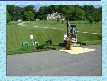
Because of the need to expose the top of the tank, we elected to use a mini excavator to handle most of the digging. These small machines have really made it so much easier to work on dry hydrants.
