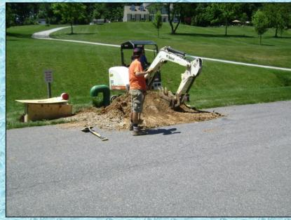
With the new suction pipe installed, the site was prepared for several days of no activity. The concern was security, vandalism, rainfall, and dirt falling in. Fortunately, the hole was less than 4-ft deep so shoring operations were not needed. A simple wooden box was built and the flanges were covered with wood blanks and dirt was backfilled in the void spots.
