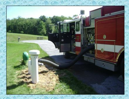
The next step in the repair process was to flow test the tank to ensure that everything worked right. Actually – given the type of damage found, flow testing could have been done before the hole was filled back in – just in case there was a problem with the suction pipe inside the tank – something that could not be seen from outside of the tank.
