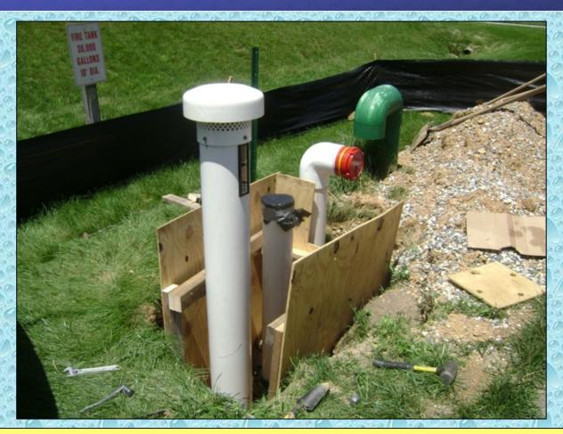
With all of the new pipes and flanges now in place, it was time to install the fill connection and then fill in the hole.
