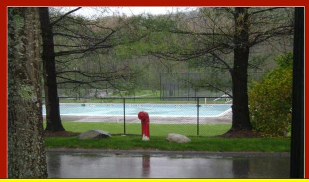
The fire protection water supply for the housing complex is the community swimming pool. It has one dry hydrant that provides FD access to the water. Hope that the homeowners know that their fire hydrants are worthless!
