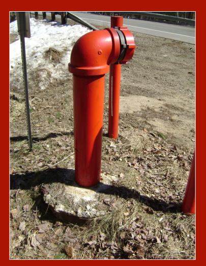
Although many DFH installations today use PVC pipe. We do like the iron pipe in terms of ruggedness – especially when having to battle snow plows along the road in the winter time.
