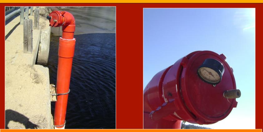
To help ensure the DFH is ready for use in the winter, the FD charges the pipe with air to prevent freezing. The gauge allows for inspection during the winter months to see if the air blanket needs boosted.
