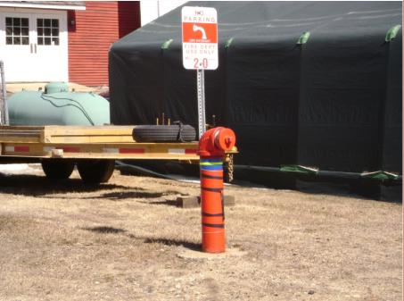
This DFH is located in the old Iron Works area of Gilmanton and accesses a pond about 75 feet off of the main road. It is made of 6-inch iron pipe and is trimmed out with a 6-inch NST male fitting.
