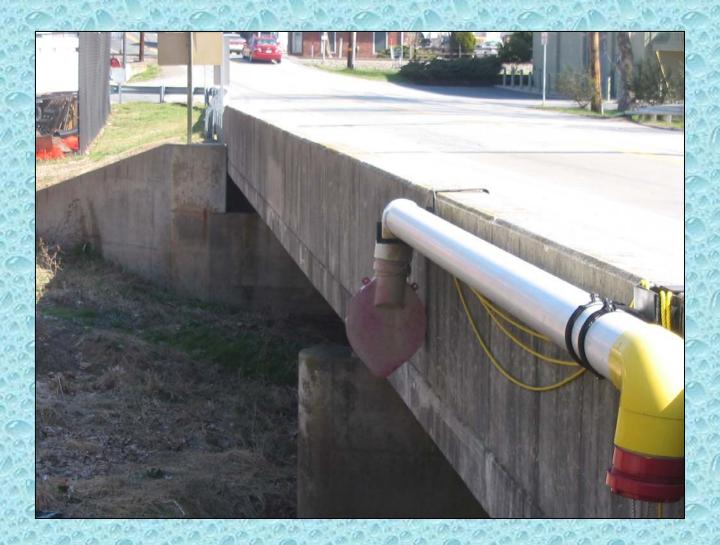
The special bridge mount was designed so that no holes were needed in the State-owned bridge.
