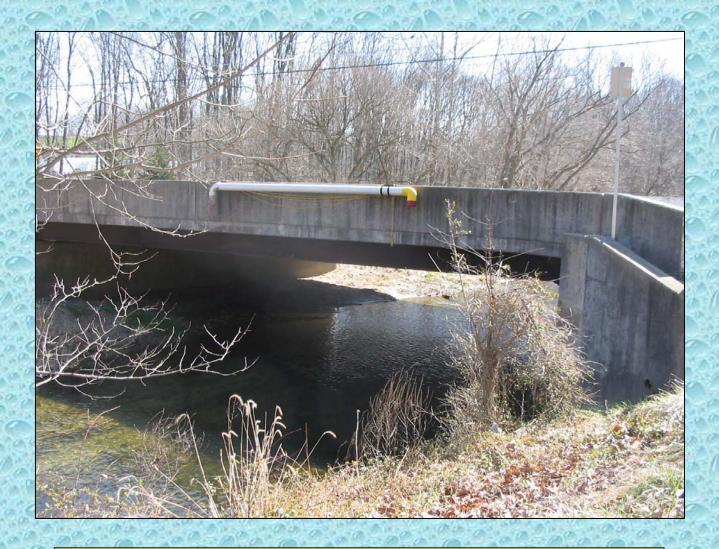
The dry hydrant at this bridge is stowed in brackets along the outside of the bridge wall. This protects the DFH from snow plow damage and allows it to be in a ready position for lowering into the waterway.
