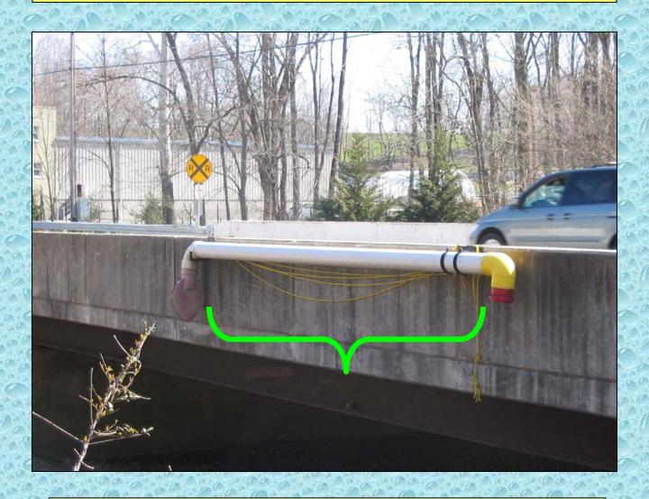
A simple, mechanical advantage system is used to lower and retrieve the DFH.
