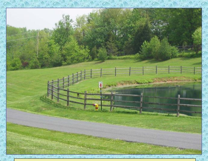
The position of the DFH allows for the easy access to suction connection – without having to deal with going under or through the fence.
