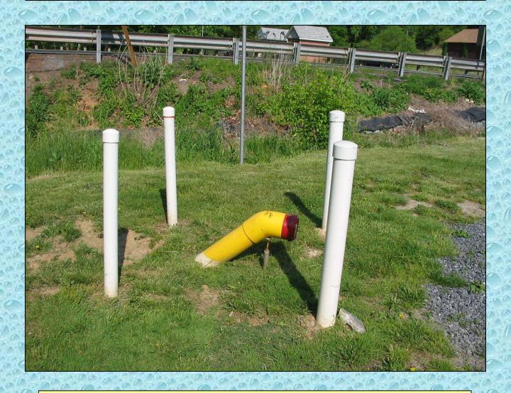
Because of the long run of pipe, a 45° degree elbow was used to help reduce the friction loss in the DFH.
