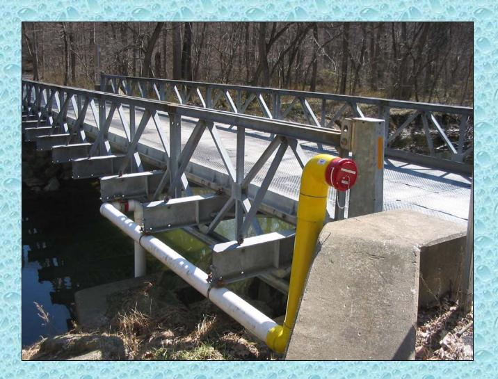
The design of this dry hydrant incorporates the use of a few simple clamps that attach the piping to the bridge supports.
