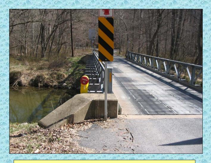
In order to access the water, a dry fire hydrant was designed and attached to the bridge so that a pumper could set up for drafting without having to worry about the weight restriction on the bridge.
