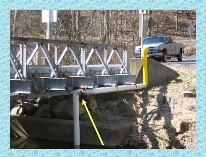
A Kochek swivel is used to allow the DFH to raised out of the water if needed.
