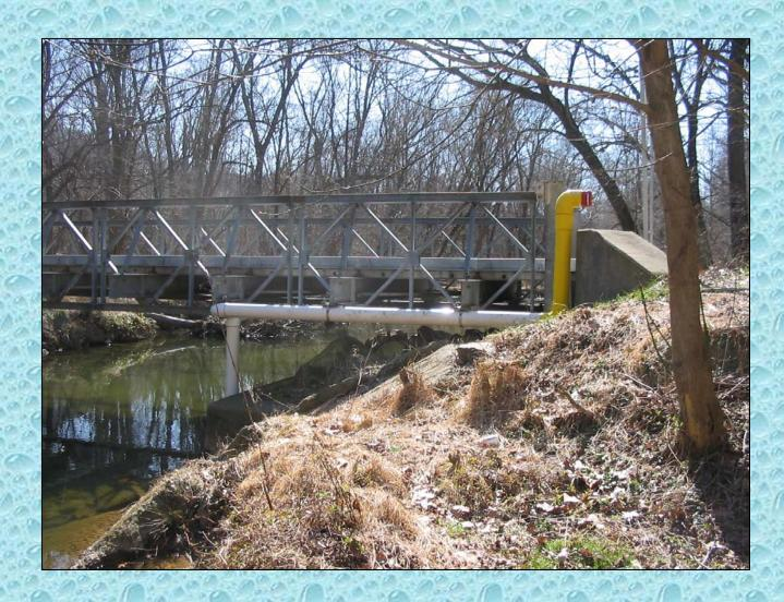
Although the run of pipe is a little long, the elevation (lift) is within reason and this DFH can support a 1,000 gpm flow.
