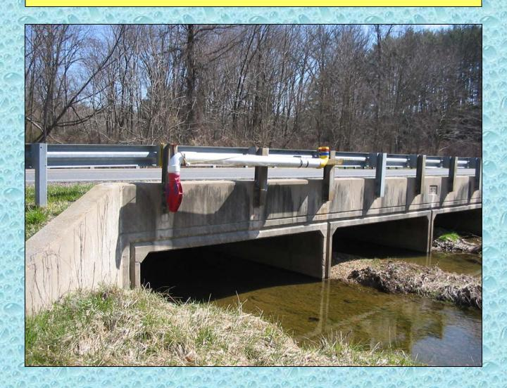
The hydrant is made of 6-inch PVC pipe and easily lowers into position. There are no swivel fittings used in this design.
