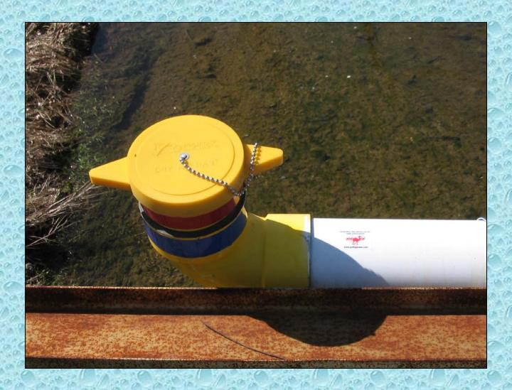
The hydrant is trimmed out with a Kochek, 6-inch male, NST suction fitting with protective plastic cap.
