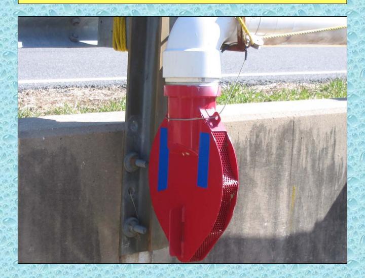
A simple pulley system is used to lower and raise the hydrant when it is needed. The hydrant is also outfitted with a Kochek teardrop strainer designed for taking suction in moving water.
