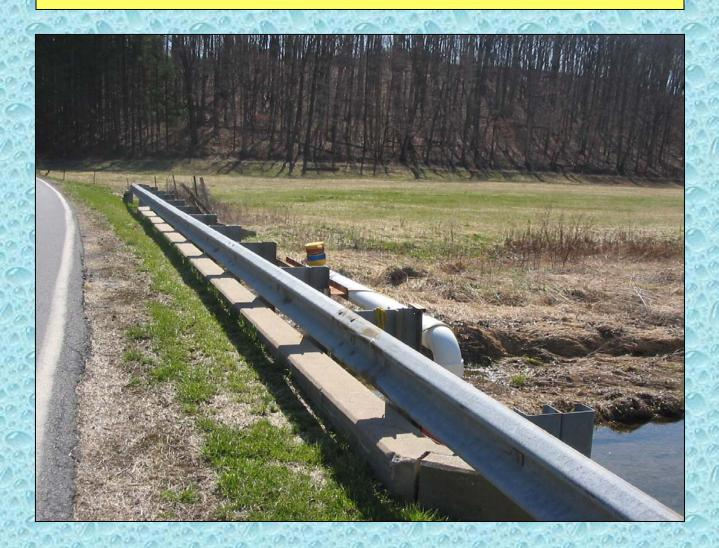
The dry hydrant is mounted to the guard rail supports which provide a stable mounting platform and protect the pipe from winter time damage (snow plows).
