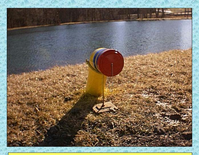
Finally, a support stanchion was fabricated and installed to help support the pipe when FD suction hose is attached to it.
