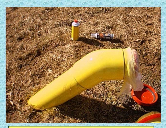
The old head was cut off below the elbow and a new elbow and head assembly was glued on. The pipe was painted yellow using UV resistant spray paint.
