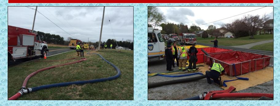
Meanwhile, back out at the rural hitch, tankers continued to pump off their water while crews worked to get a dump tank operation up and running. Around the 45-minute mark flow was moved to 1000 gpm using the rural hitch.
