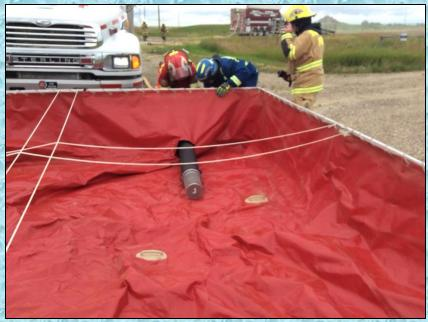
Crews work to get the first dump tank (3000-gal) set up for a load of water. A barrel strainer was used because it was the best performing strainer available.
