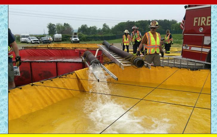
By the 39-minute mark, three dump tanks were now in operation as were two jet siphon-style water transfer devices.
