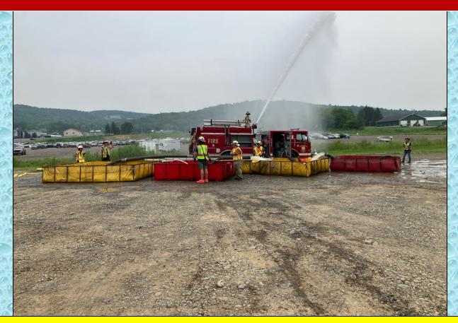
A four-dump tank arrangement was the final layout that supported a peak flow of 1663 gpm!
