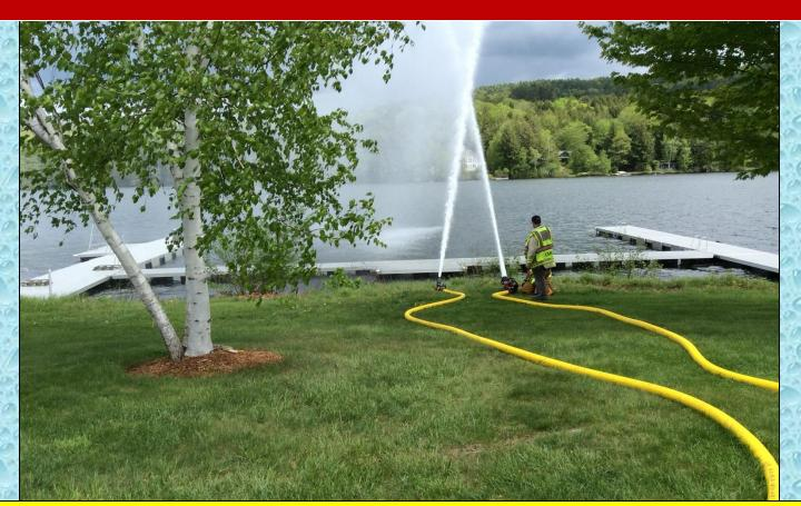
Two, ground-based monitors were used to discharge water back into the lake. Fairlee Engine 5 supplied both monitors.
