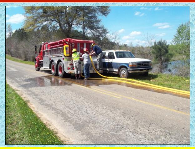
After the first tanker was filled and sent back to the dump site, the crew then worked to set up a 5-inch LDH line in order to create a second fill station.
