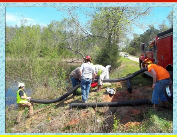
Because the performance of the dry hydrant was suspect, the crews decided to go the traditional drafting route and put suction hose into the water.
