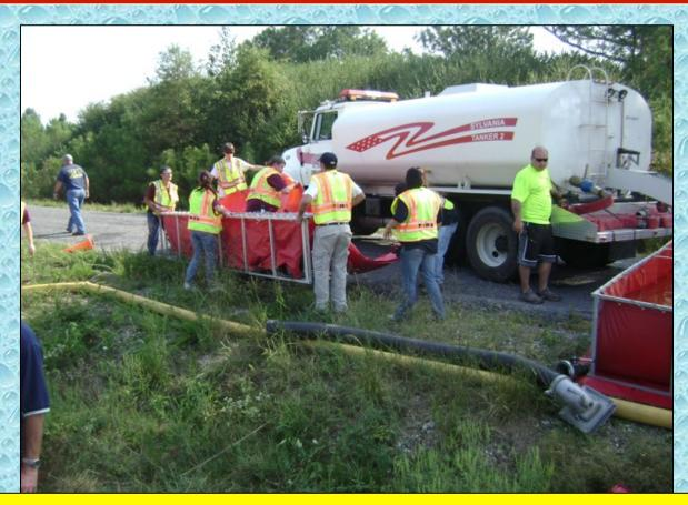
A second, 3,000-gallon tank from Crossville Engine 6 is shown being set-up above as the crews work to build out a dump site capable of handling 500 gpm at the 15-minute mark.
