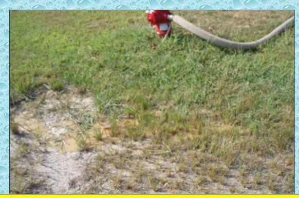
One problem that arose during the operation was that no control valve was placed on the hydrant. The hydrant had to be opened and closed as needed to fill the tank - which caused the hydrant drains to discharge water thus causing water to bubble up through the ground. An external valve should have been used on the hydrant – it would also have made for less work when opening up to fill the dump tank.
