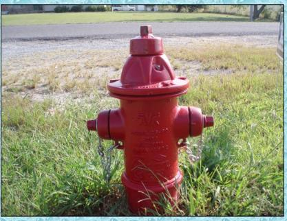
This hydrant on Buttrams Crossing Road had been used in previous year's drills. However, the flow rate had been below 1,000 gpm both times — more like in the 600 to 750 gpm rate. The problem posed for the 2010 drill was the ability to fill tankers using this hydrant at a rate high enough to support the fire attack operation. And...this hydrant presented the shortest water hauling distance for the 2010 drill, so it was an attractive site.
