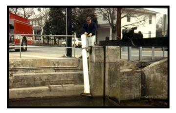
The mounting bracket and a rope allows the suction pipe to be raised so strainer can be cleaned if needed.
