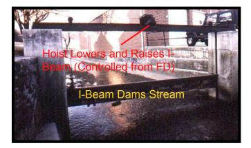
The arrangement consists of an electric hoist controlled from within the fire station and an I-beam that actually dams the stream
