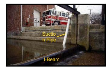
When the I-beam is in place, the stream is deep enough to allow drafting with a pumper.
