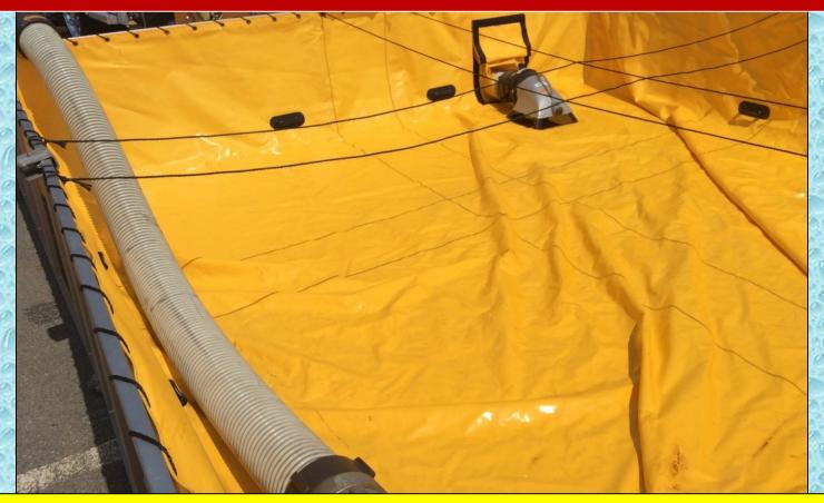
One of the suction lines was deployed through the drain sleeve and one was deployed over the tank frame..
