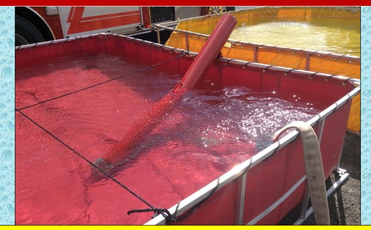
A Holley Transfer Pipe was deployed as the first water transfer device. However the distance between the two tanks proved problematic and a traditional suction hose jet transfer arrangement replaced this set-up.
