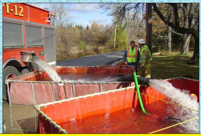
A good example of dumping and transferring water. The level in the drafting tank shows that this operation might be approaching its maximum capability.
