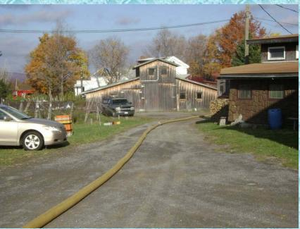
E16 lays 1,000 feet of 5-inch supply line through the complex. The ability to get this smaller engine into position in this type of complex and then supply it with LDH allows a crew to mount a large caliber fire attack without the need for multiple supply lines.
