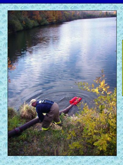
Initially, 20-ft of 6-inch suction hose was used to reach the water. This was changed when the relay operation began due to concerns over vegetation possibly clogging the strainer.
