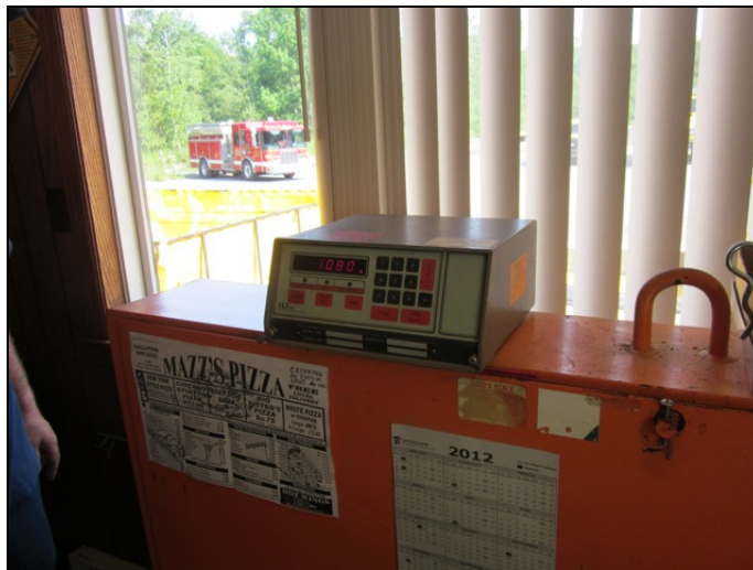
Figure 23: Scale readings were displayed digitally inside the scale house and were recorded in an Excel spreadsheet for later analysis.
