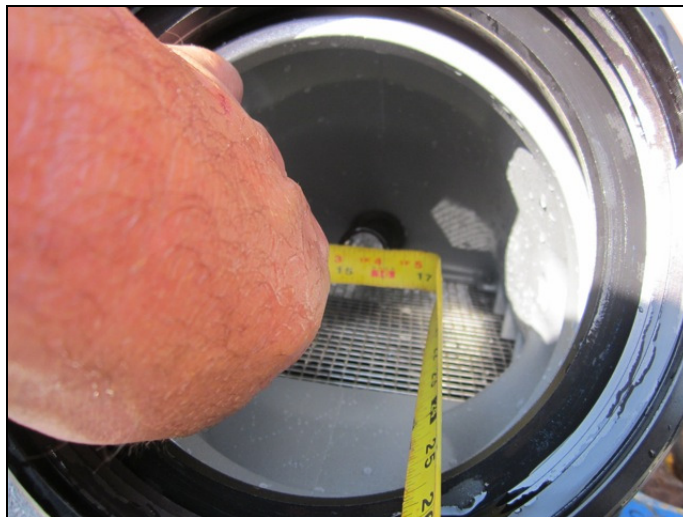
Figure 9: The TFT strainer had a 1-inch discharge orifice.
