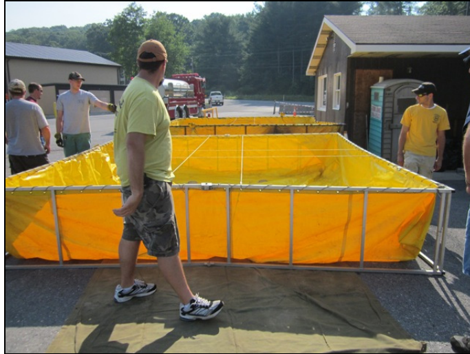
Figure 22: With the Collection Tank in position on the scale, the 3,000-gallon Supply Tank (foreground) was placed.
