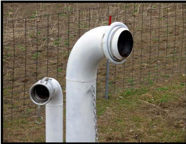
The 6" suction pipes are equipped with irrigation type connections to facilitate quick and easy suction hose hook-up.
