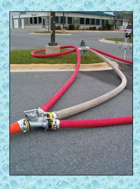
This layout maximizes the available water from a fire hydrant by getting big lines on each outlet.
