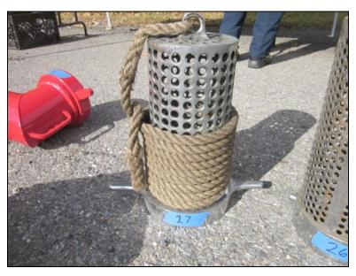
Figure 39: Barrel Strainer (Manufacturer and model unknown – possible Seagrave). The strainer came from a 1959 Seagrave pumper and had approximately three hundred ninety-two,  $\frac{1}{2}$ -inch holes – some of those holes were in the end of the strainer. The holes all had smooth edges.
